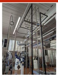
Valve Clusters: designed by Phoenix Welding, enabling simultaneous, timed filling, emptying, and cleaning of production lines without the possibility of mixing. To address the needs particular to your industry, we can design valve clusters.
